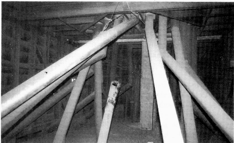
Spout area below headhouse
