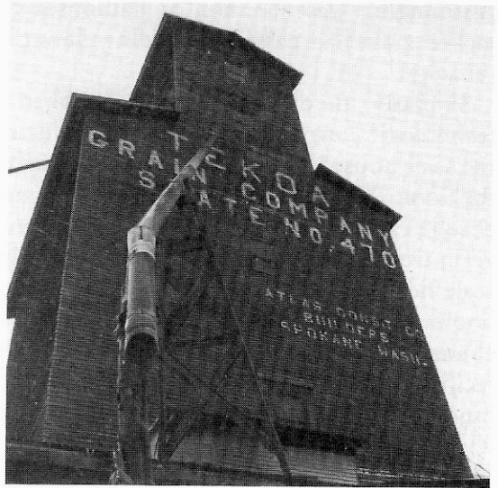
Distributing spout, with spout holes
