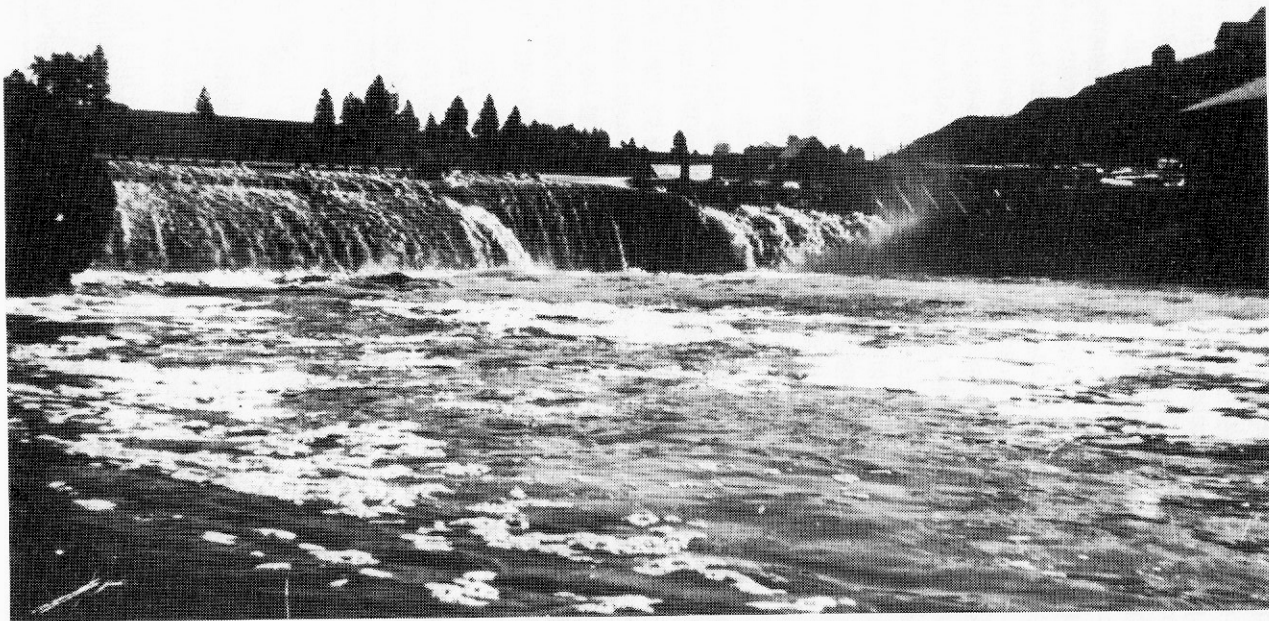
Water flooding over the large mill dam at the east end of Palouse.
