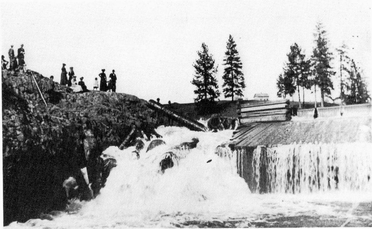
Here, a log jam can be seen forming in the spillway.
