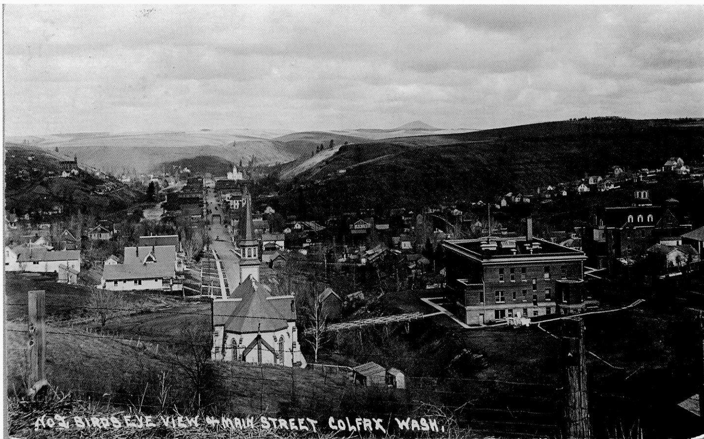
Panorama taken from south hill looking directly down Main Street This clearly shows the relationship of these three Catholic structures on the south edge of Colfax.
