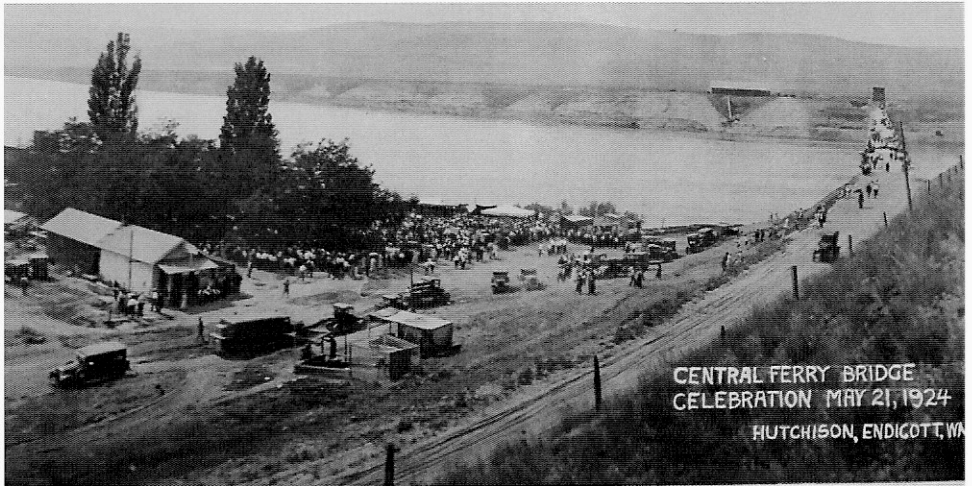
Central Ferry bridge on the Snake River (1924)
