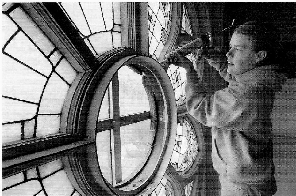
Geoff Crimmins, Daily News , April 9 and 10, 2005 Restoration work in progress, 2005
