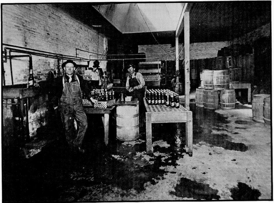
Palouse Brewery Bottling Plant
