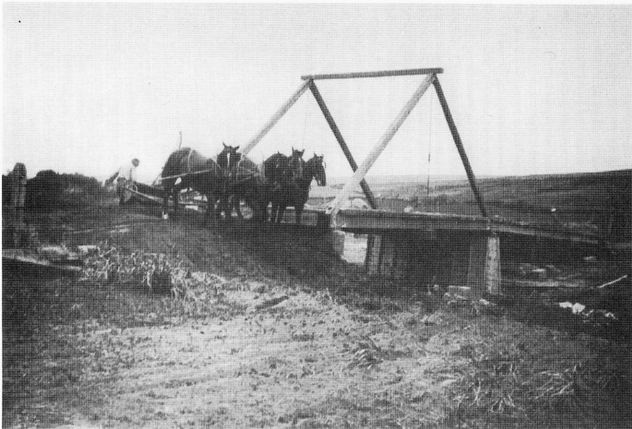
Smoothing out the bridge approach, Roy Davis driving.
