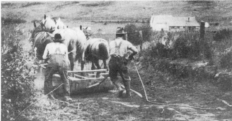
Grading the hill (L. to R.), Orrie Hatley and Roy Davis.
