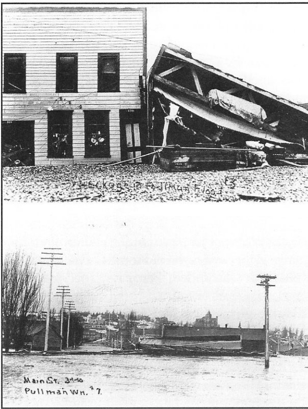
March 1, 1910 flood at Pullman, with bottling works buildings in foreground. —Washington State University Libraries
