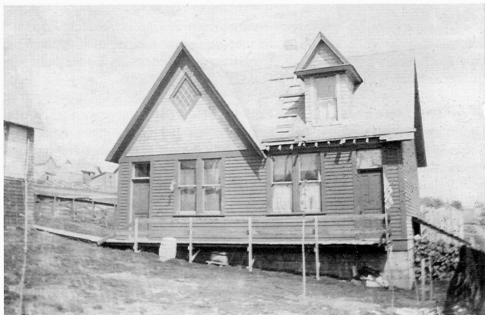
The Parish House, 1898. Built in 1891 this served as the vicarage until 1919, after which it became the Parish Hall until destroyed by fire in 1926.
