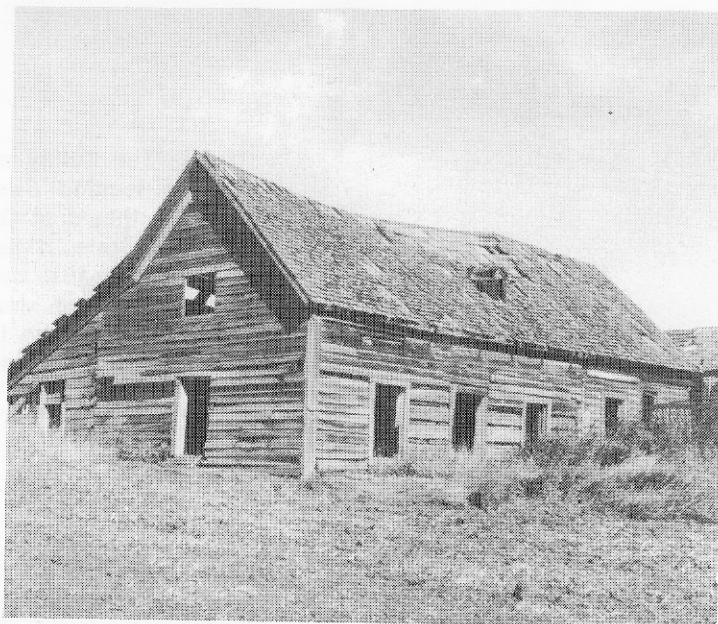
This cabin was built by Thomas Shoffen in 1875. It can be seen from highway 195 just north of Uniontown in a field to the east. It was later sided with sawn lumber from the Palouse mill.
