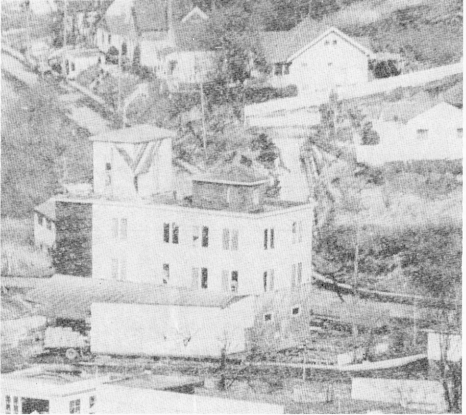
The last Colfax Flour Mill building. Picture taken 1955 courtesy Colfax Gazette.
