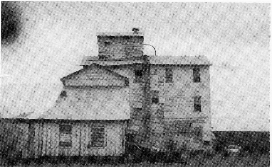
The LaCrosse Flour Mill building
