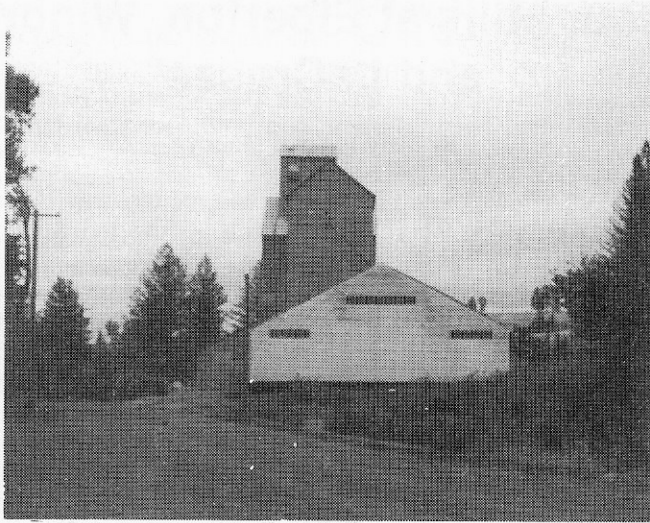
The Elberton Flour Mill building at new location.
