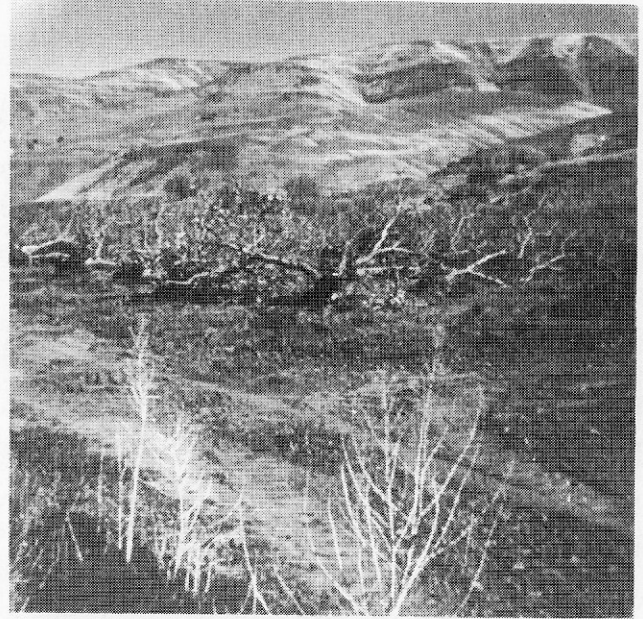
One week later they are pulled for Lower Granite Dam Project
